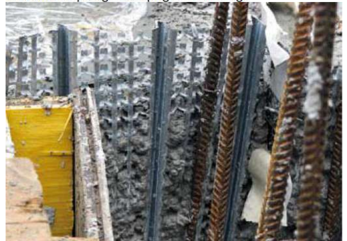
Meshes well with High-RIP® when creating permanent formwork. Preparation of the areas (forming) in one go.
