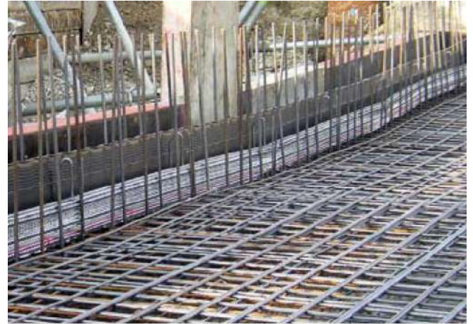
Upturn of joint strip for water sealing on a floor surface. High-RIP® is self-stiffening thanks to the longitudinal ribs and thus helps against upright armouring.
