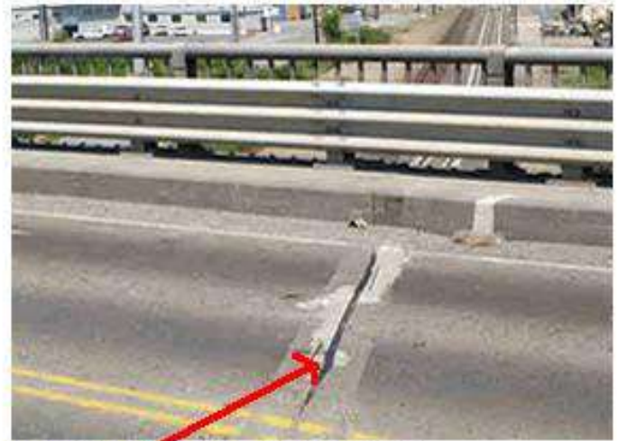
JOLLY BITULEX EXPANSION JOINT FILLER IN BRIDGE
